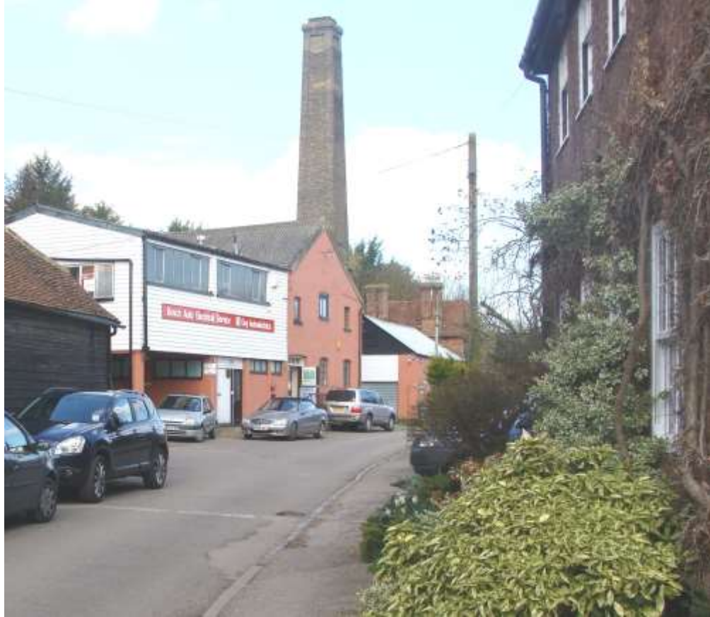
Picture 7- Distinctive chimney, Mill End.
