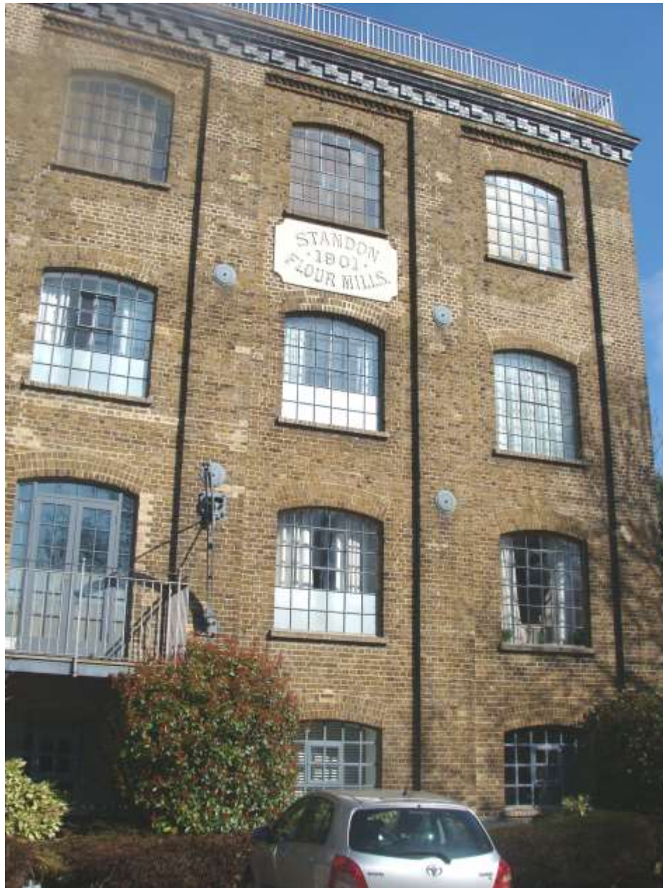
Picture 6 – The sensitively converted Flour Mill.
