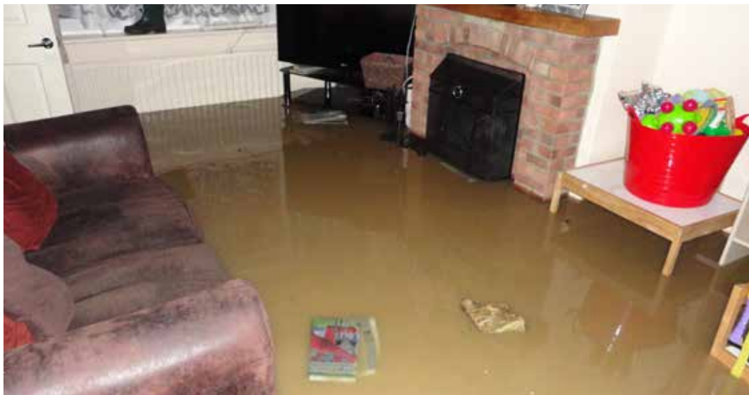
Local Flooded House
