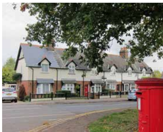
Typical terrace in Puckeridge
