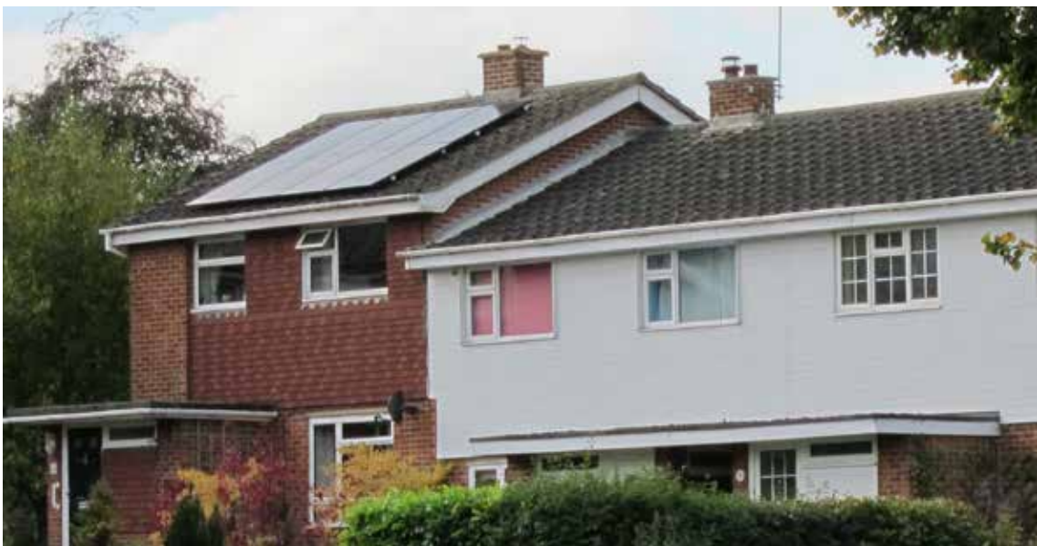
Local House with solar panels
