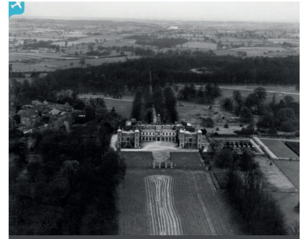
Figure 3.9 Aerial Photograph of Hatfield House, looking north, 1948. Source: Britain from Above
