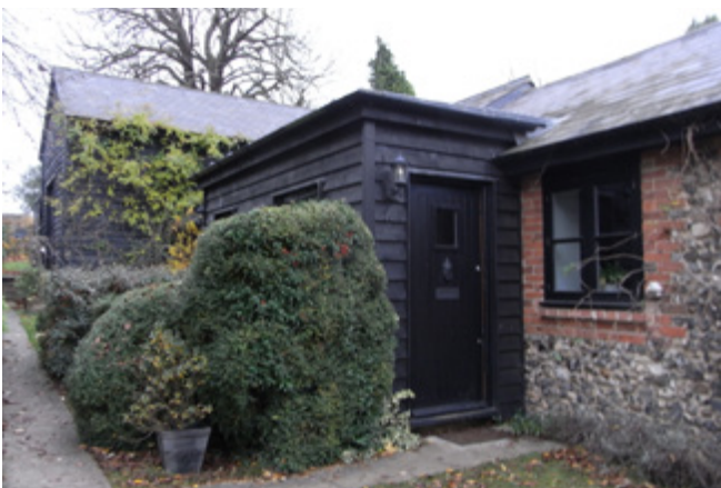
Barn Conversion – Green End
