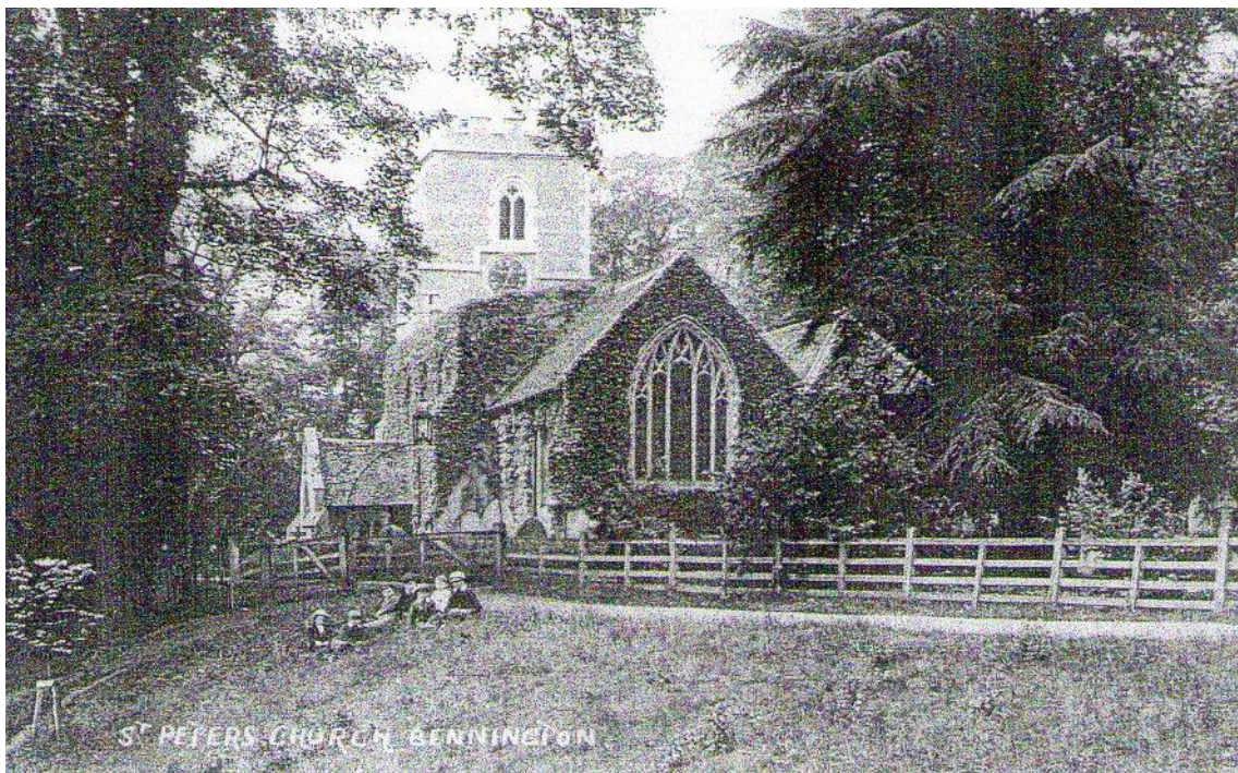
Picture 1. Church of St Peter Bennington - date unknown probably late 19 th early 20 th century. Church interpreted as being covered in vegetation; fence no longer in place, neither is semi circular metal structure appearing to support a lantern. Reproduced courtesy of Hertfordshire Archives and Local Studies (HALS).
