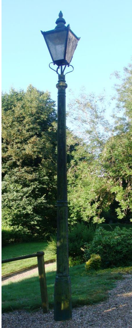
Picture 20. Cast iron lamp on tapering octagonal column probably of late 19th century date.
