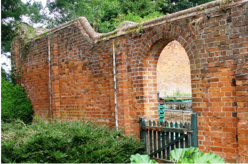
Picture 18. High quality wall enclosing western side of Kitchen Garden.
