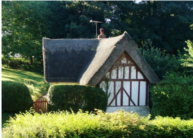
Picture 4. Unusual 17th century single storey thatched property with later fake timbering applied.
