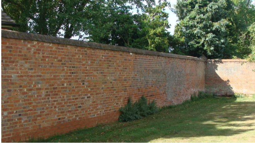
Pictures 31-33. Former kitchen garden at Bury Lodge Farm. Top traditional box edgings which the owners are encouraged to retain. Below walls about 3m in height, some repairs desirable. Grant assistance may be available.
