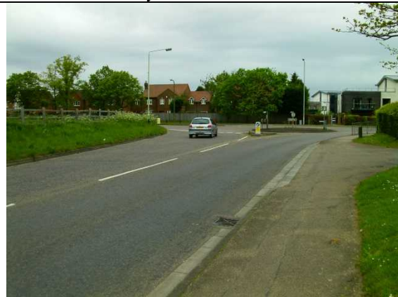
Image 3: Thieves Lane approach to roundabout
