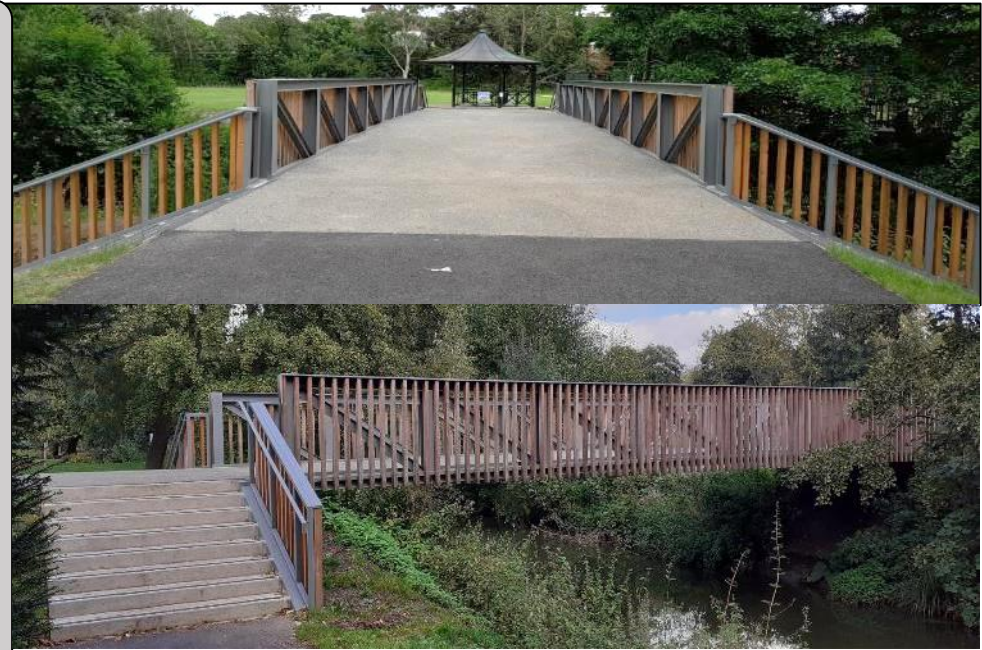
The new, wide, accessible and attractive bridge connects the events areas and the children's play spaces.
