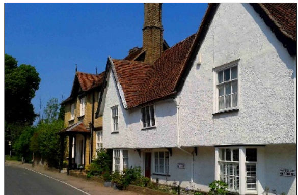
Jettied house with handmade tile roof
