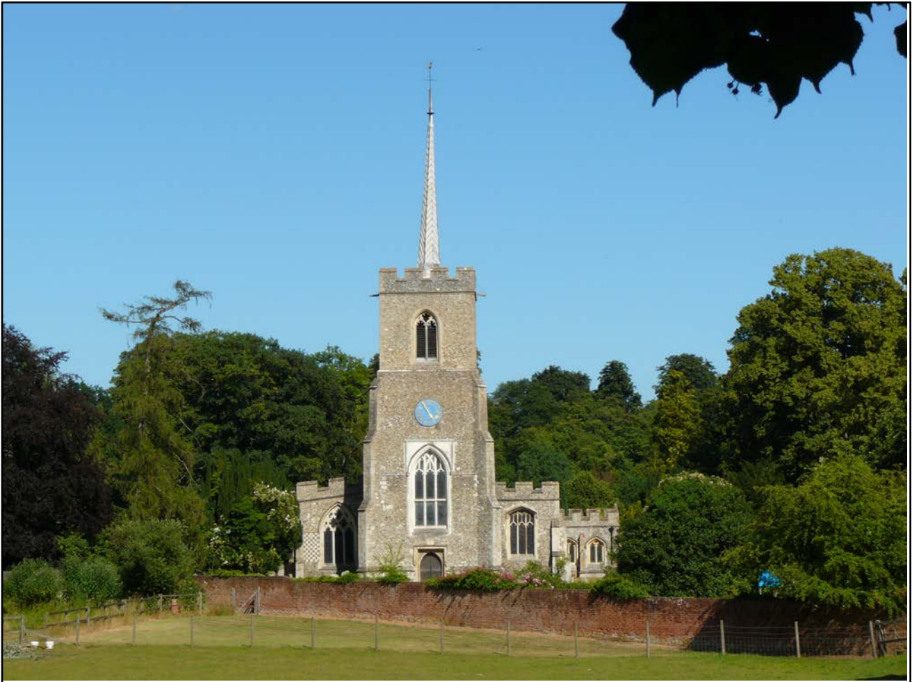
V1: St Andrew's Church from gate by bus shelter on B1004
